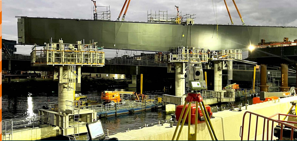
Live survey monitoring during installation of steel girder
